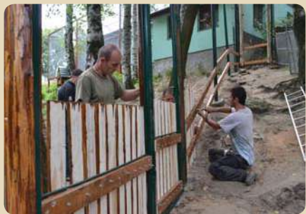
Rekonštrukcia plotu pre kozy kamerunské Reconstruction of a fence for Domestic Pygmy Goat
