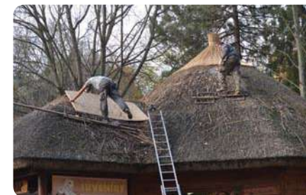
Oprava strechy ZOOshopu Repairing of the ZOOshop roof
